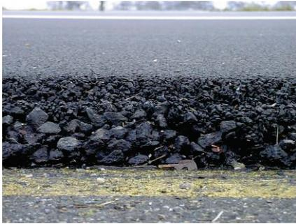
**Figure 7:** Double layer porous asphalt has a top layer, 15 – 30 mm thick, with small stones ( $\leq 8$  mm), and a bottom layer, 30 – 60 mm thick, with larger stones ( $\leq 16$  mm)
