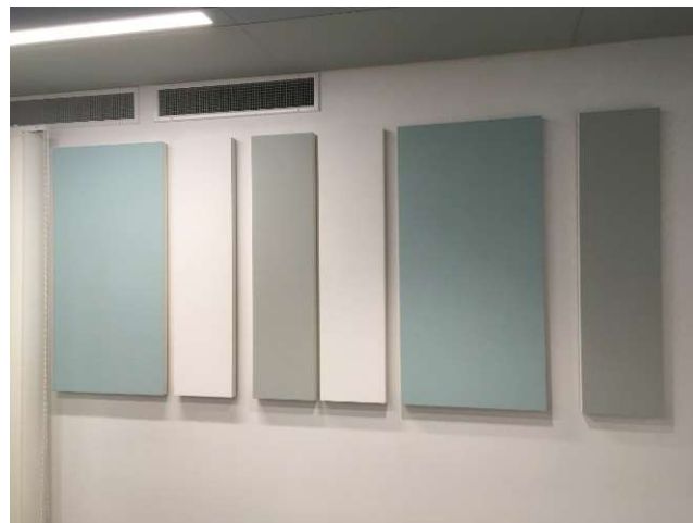
Figure 6 – Config. 4. Six vertical wall absorbers at the front on the left wall as shown in Figure 5.
