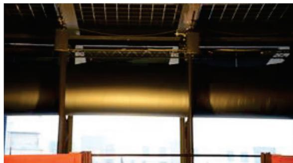
Figure 14 – As any other membrane absorber, the tube is most effective in high sound-pressure zones. *Kraftwerk* concerts, Neue Nationalgalerie, Berlin 2015
