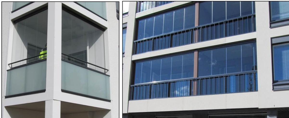
Figure 1 – Typical Finnish balconies where the upper portion of glass is made of openable panes (glazing). The lower part is usually made of larger non-openable glass panes (balustrade).
