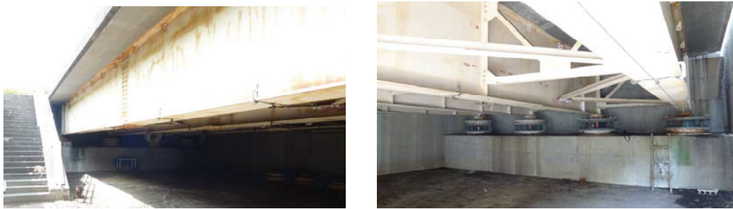
Figure 2 – Clearance under bridge
