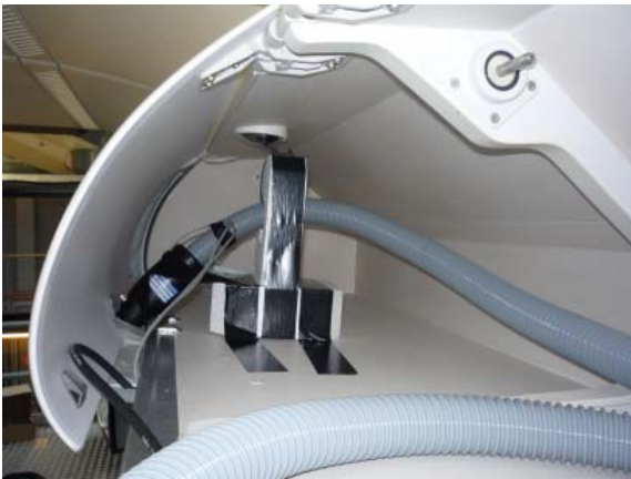
Figure 4: View into hat rack with mounted velocity measurement adaptor and extension hose of a volume velocity source.
