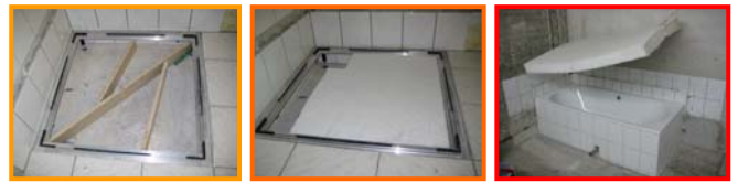
Figure 9: Test set-ups for the results in Figure 8: gap division (yellow, left), porous absorption for damping of the airborne sound field in the gap (orange, middle) and absorbing shield above the sanitary object (red, right).
