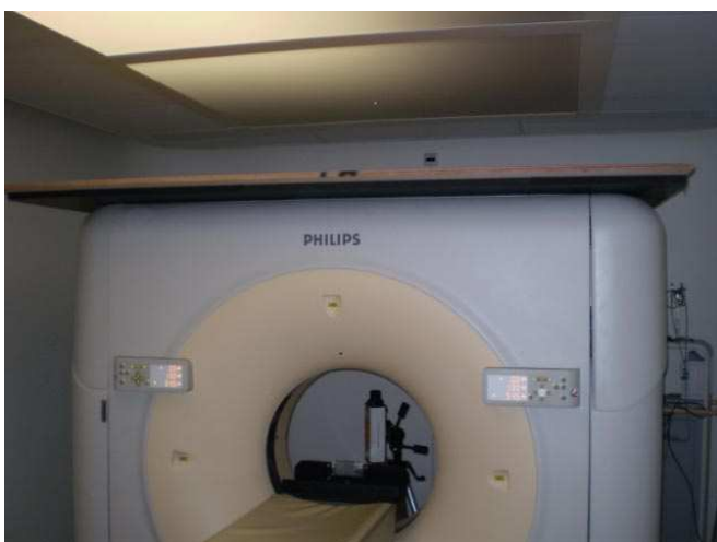
Figure 11: Plywood plate with absorbing foam lying on gantry
