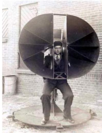
Figure 7: Sound locator Waalsdorp.
