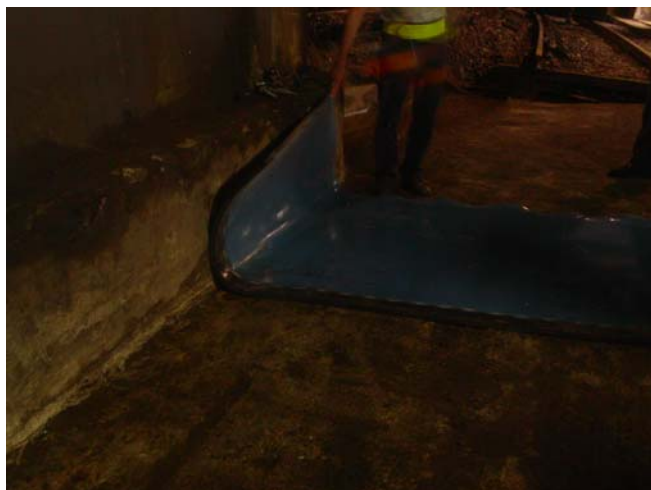
Figure 4: The resilient mat by Sylomer glued to the floor and lower walls of the tunnel.
