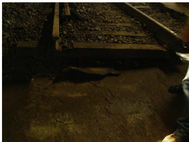
Figure 3: Cross section of the trackwork showing the larger than usual ties thinned on one side.
