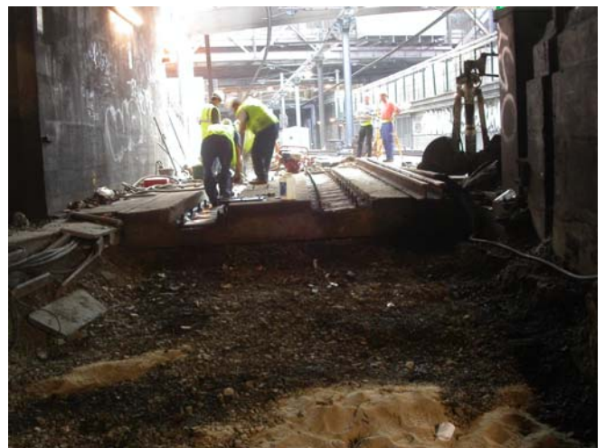
Figure 2: Entrance to the tunnel under the building; note the concrete structure in the background.
