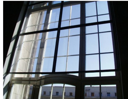
Figure 6: "Aula", absorbers made of micro-perforated acrylic glass in front of the windows.
