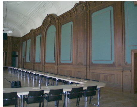
Figure 7: "Eichensaal", Broadband Compact Absorbers behind the fabric lining of the side wall.
