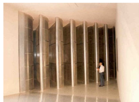
Figure 3: View to one corner of the AUDI aero-acoustic wind tunnel with BCA modules as splitter silencers [5].
