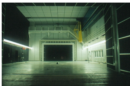
Figure 4: View from the collector to the plenum of the DaimlerChrysler aero-acoustic wind tunnel at Detroit.
