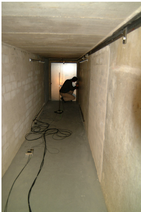
Figure 4: View into the impedance tube with 1.6 x 1.2 m cross section.
