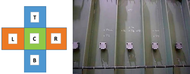
Fig 6: Arrangement of points for hammer-impulse test for measuring mode-shapes and their corresponding natural frequencies on tank walls
