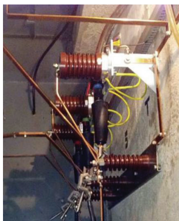
Figure 3 – Mounted couples inside a generator pit (source sparks instruments)
