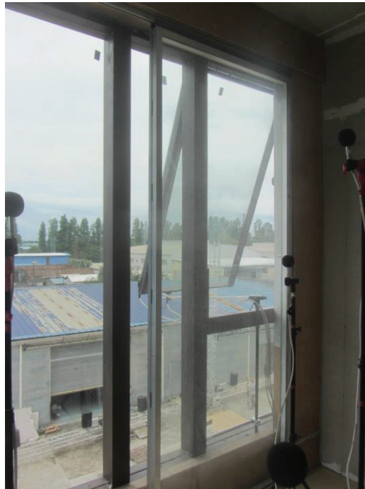
Figure 3 The view of window 3, a top hung plenum window, from inside
