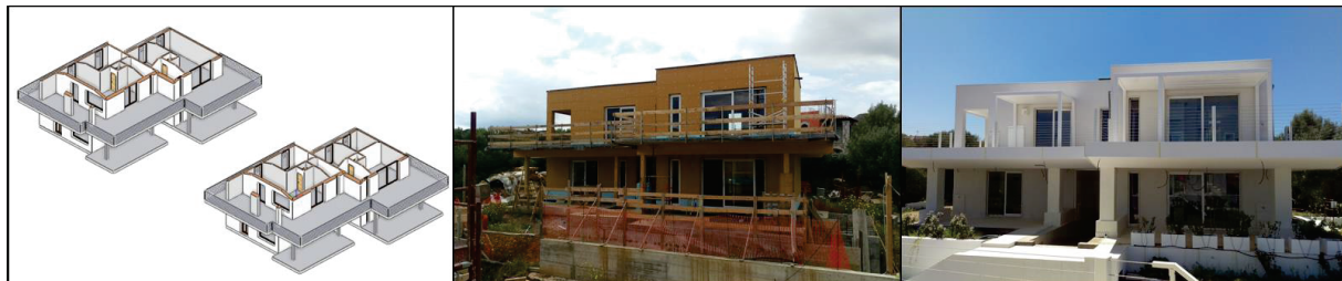
Figure 5 – case study 1 in steps: architectural BIM model, construction phase, work completed
