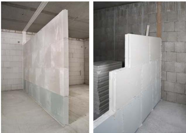
**Figure 1:** construction of gypsum walls in buildings
